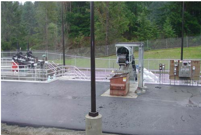
New headworks equipment at the wastewater treatment plant
